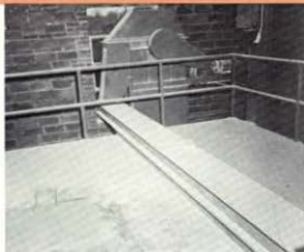
Top of huge lime storage bin which is ventilated by one of the Dustubes.
